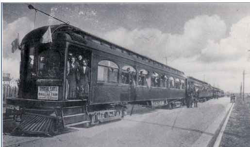
Texas Traction Company entering Dallas 1909 (left)
